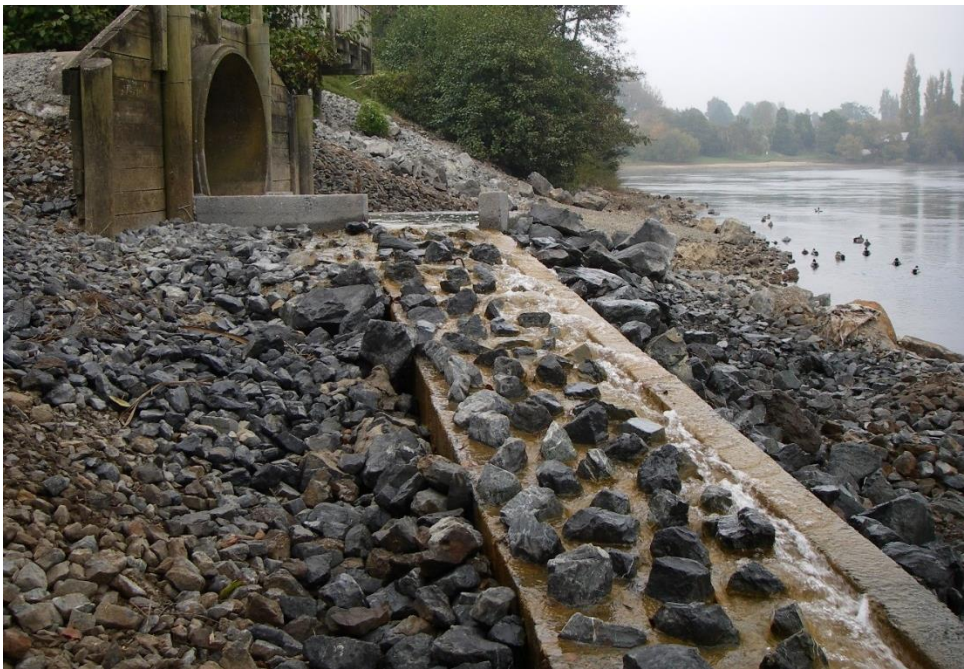
Figure I-14: The receiving pool and fish ramp operating under summer low flow conditions.
