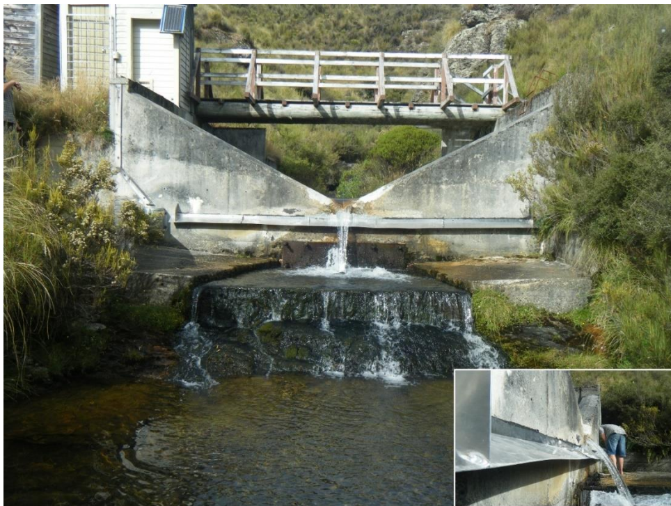
Figure 6-6: Built barrier installed in an un-named tributary of Upper Waipori River. The objective was to prevent trout and kōaro access to a key dusky galaxias stronghold in Otago. Inset shows a close-up view of the successful kōaro lip barrier. Credit: Josh Tobak.
