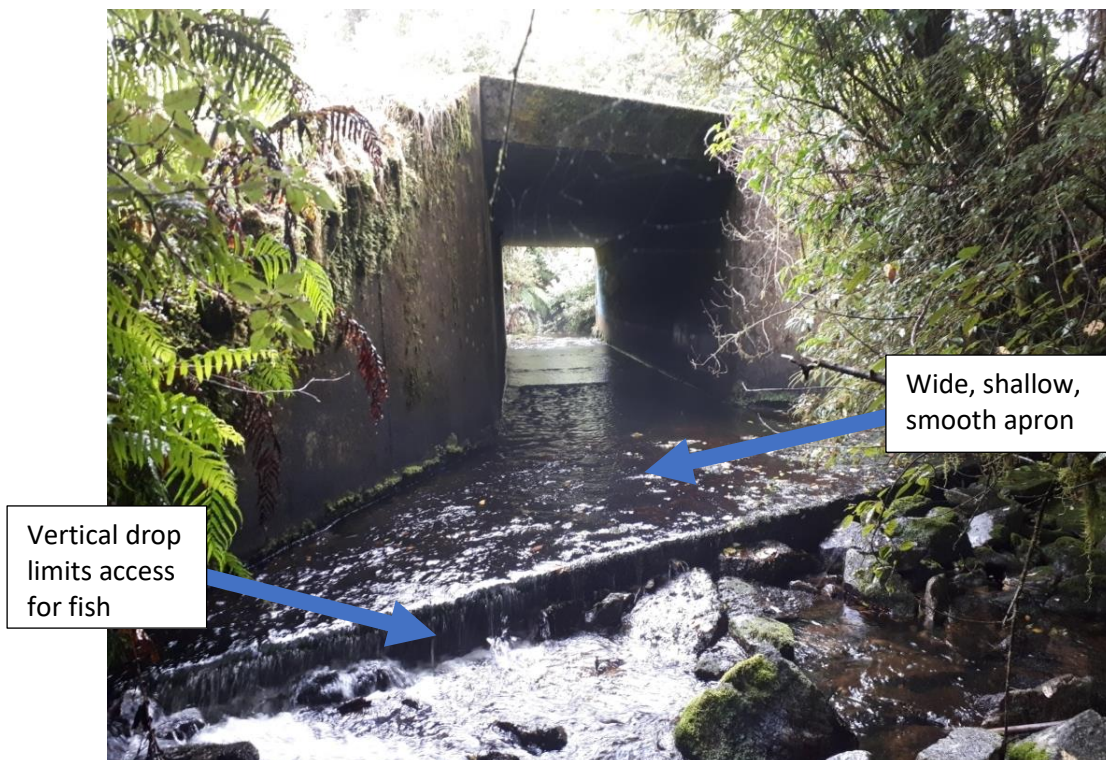
Figure E-17: Fish movements will be impeded by the fall at the downstream end of the apron and shallow water on the apron. Credit: Sam Ammon.
