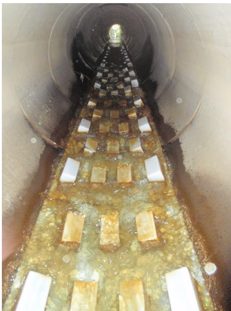
Figure 5-7: Spoiler baffle sheets installed inside a culvert.
