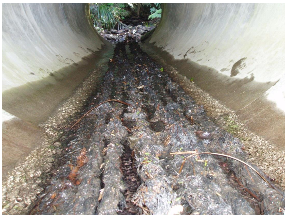
Figure 5-10: Example of good mussel spat rope installation showing fish 'swimming lanes' between ropes. Note that the number of ropes has been scaled up to match the size of the culvert. Photo: Bruno David.
