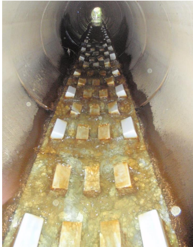
Figure I-15: The culvert barrel following installation of the spoiler baffle sheets.
