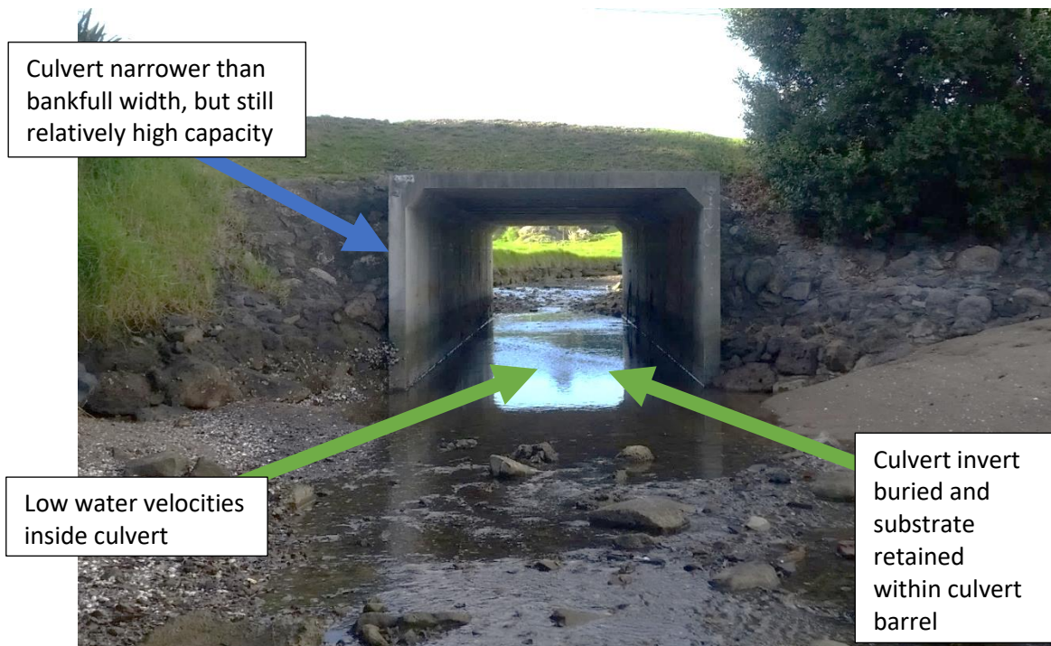
Figure E-22: Example of a culvert in a tidally influenced area. The culvert invert is embedded meaning that natural substrate is retained through the culvert. Culvert width relative to the stream bankfull width is lower than recommended, but because the culvert is in a tidal area, low water velocities will exist through the culvert during slack tide conditions. Credit: Bryn Quilter.
