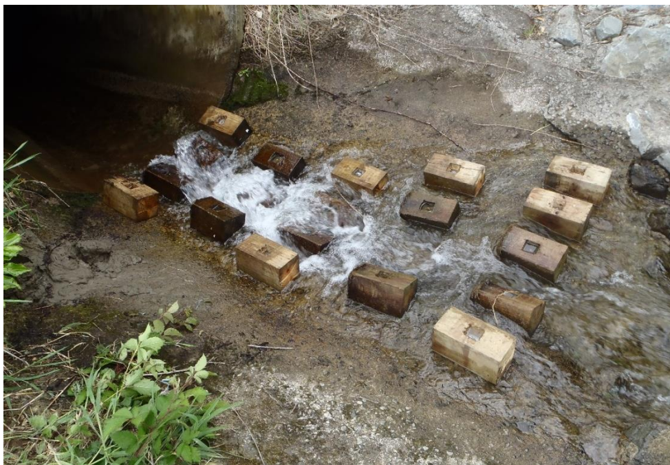
Figure I-13: Rectangular spoiler baffles anchored to the Upper Kingston Road culvert apron.
