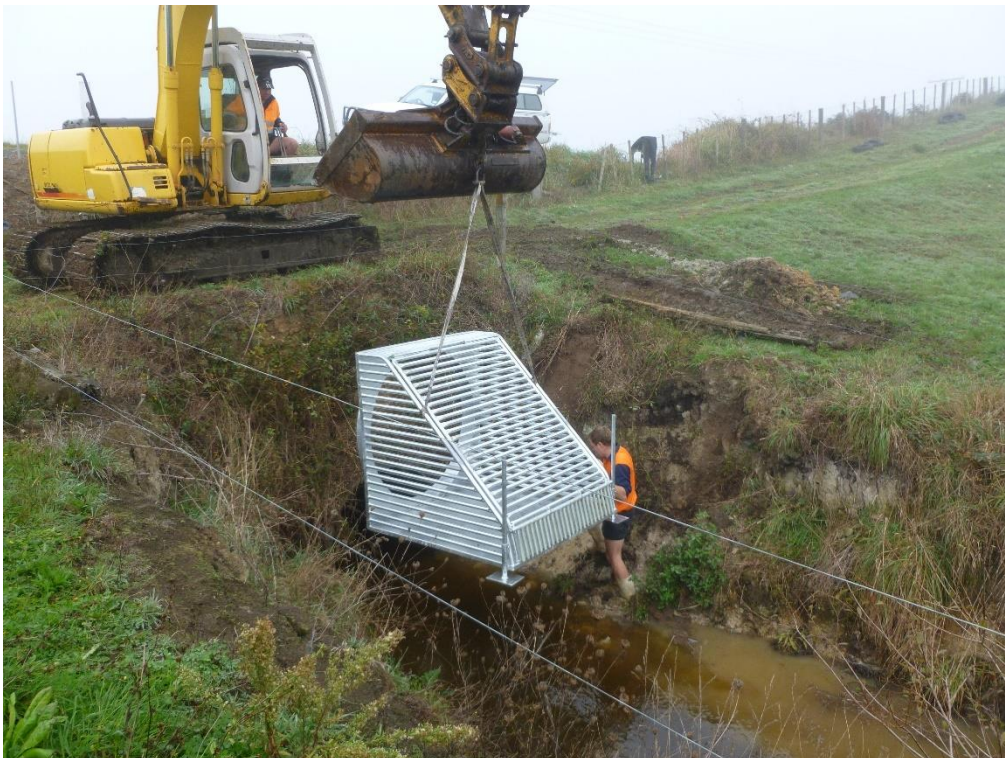
Figure 6-8: One-way gate structure prior to installation showing screen that can be lifted for inspection and clearing of debris. Credit: Adam Daniel.
