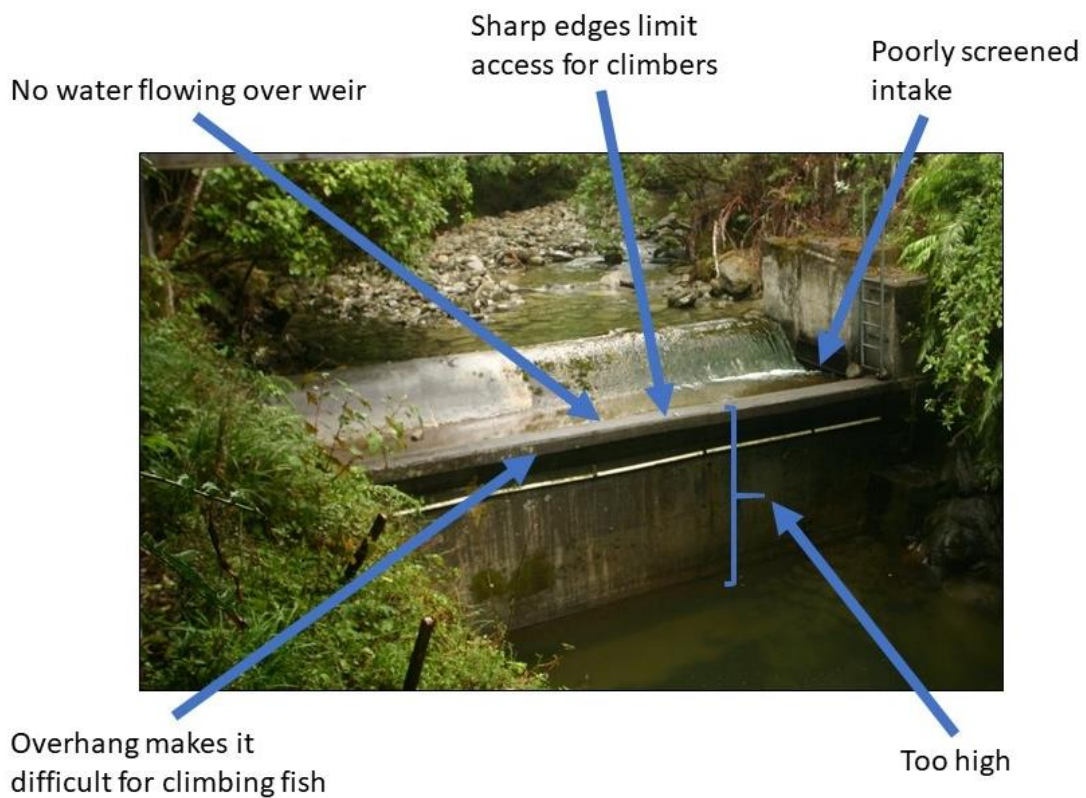
Figure 2-3: An example of an intake weir identifying features unsuitable for fish passage.
