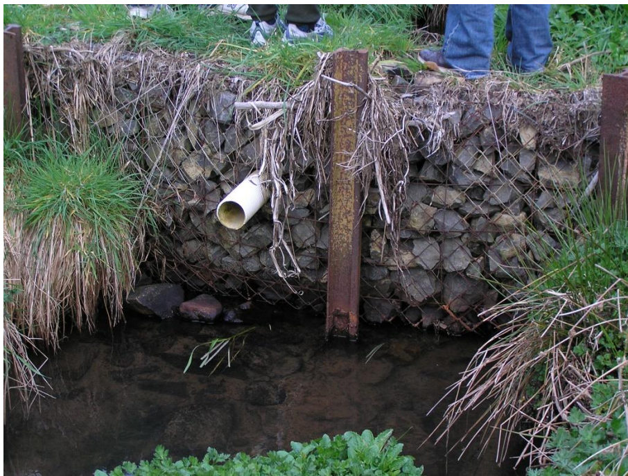
Figure 6-11: An unsuccessful gabion basket weir installed to allow migratory native fish access, while preventing trout access in Orokonui Creek, Otago. Credit: Sjaan Bowie.
