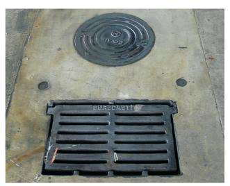
An oil/water separator for stormwater treatment
