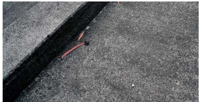
A low nib wall or speed bump is all you need to keep contaminants out of stormwater
