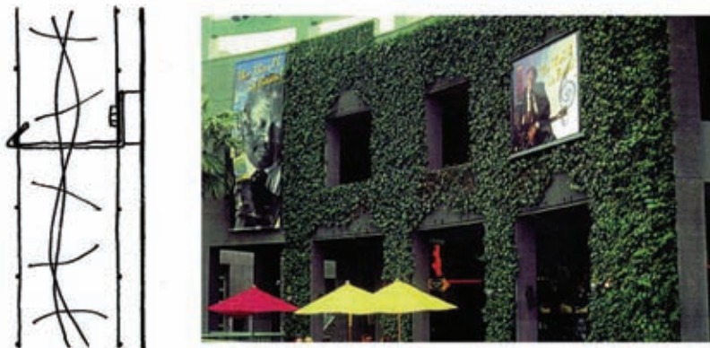
Figure 9: A greenscreen (left) with the two meshes hung on the solid façade
