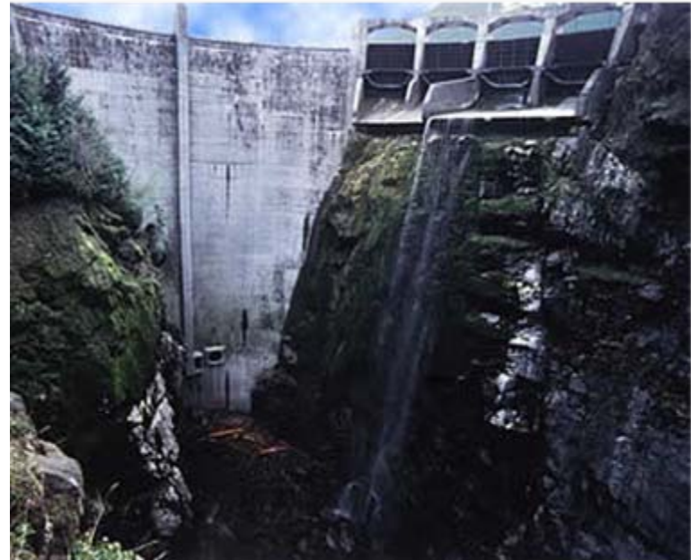
Glines Canyon Dam – 13.3MW, 65m high. Elwha River, WA
