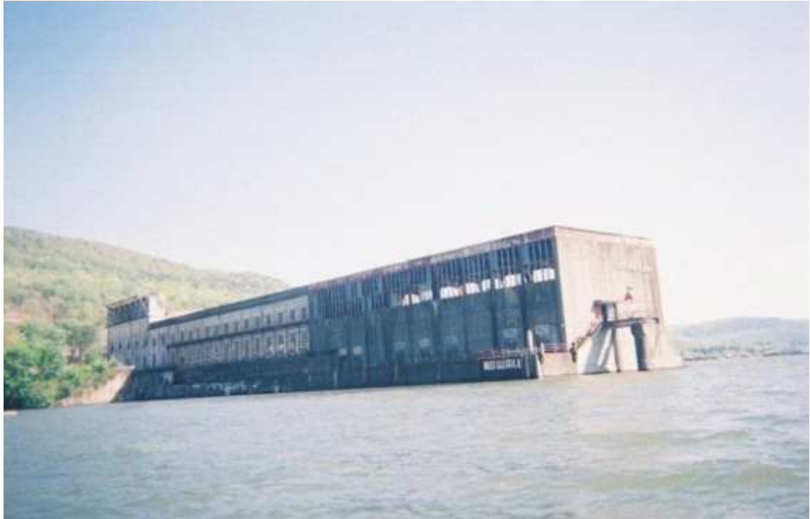
Remnant of the dismantled Hales Bar dam, Tennessee River.
