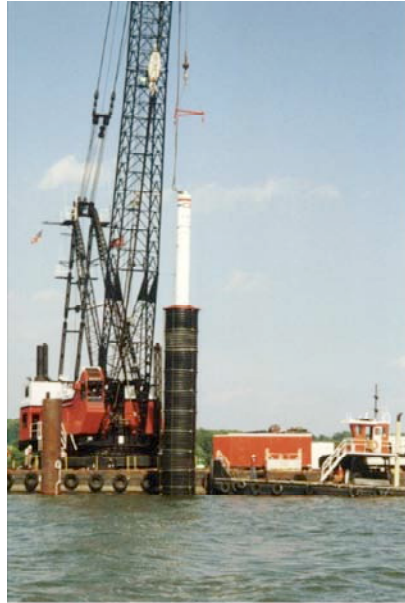
Figure 3.2: Sound Dampening During Pile Driving
