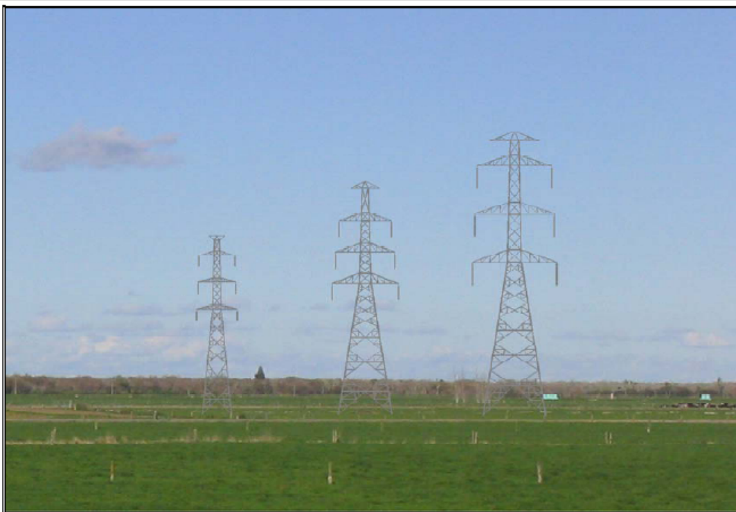
Figure 11 – Comparison of typical tower height suspension towers for 220kV, 220kV alternative, and 400kV Proposal typical tower heights (impression only)
