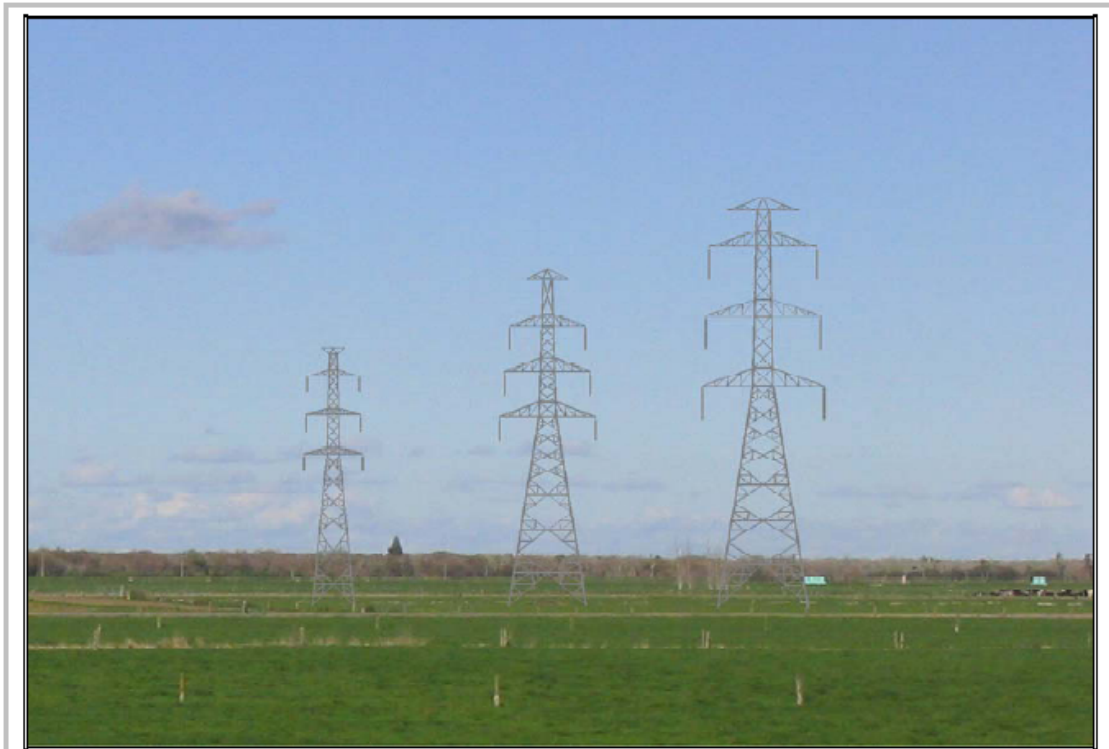
Figure 11 – Comparison of typical tower height suspension towers for 220kV, 220kV alternative, and 400kV Proposal typical tower heights (impression only)
