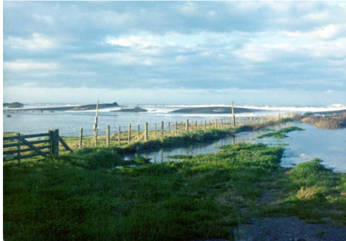
Figure A3.1: Waves overtopping the shingle/sand barrier at East Clive, south of Napier, during a storm in August 1974. [Source: Ministry of Works and Development collection, Napier.]
