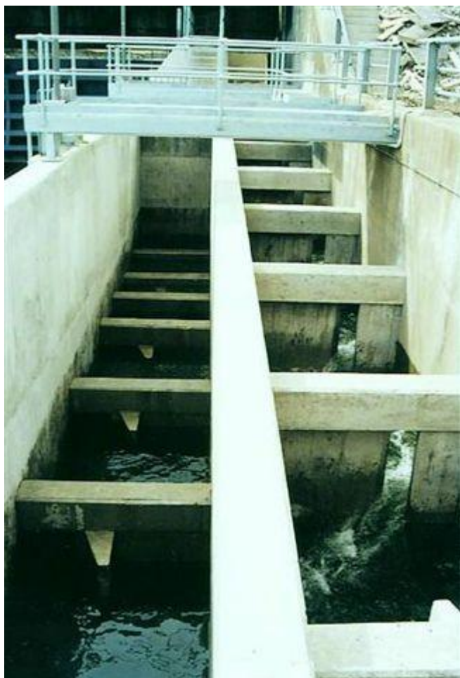
Figure 24. The fish pass on the Mararoa Weir in Southland where trout have been trapped negotiating the pass.
